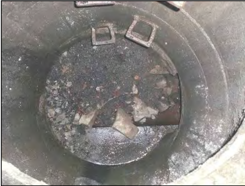
Bauschutt [Backnang, 2014]
