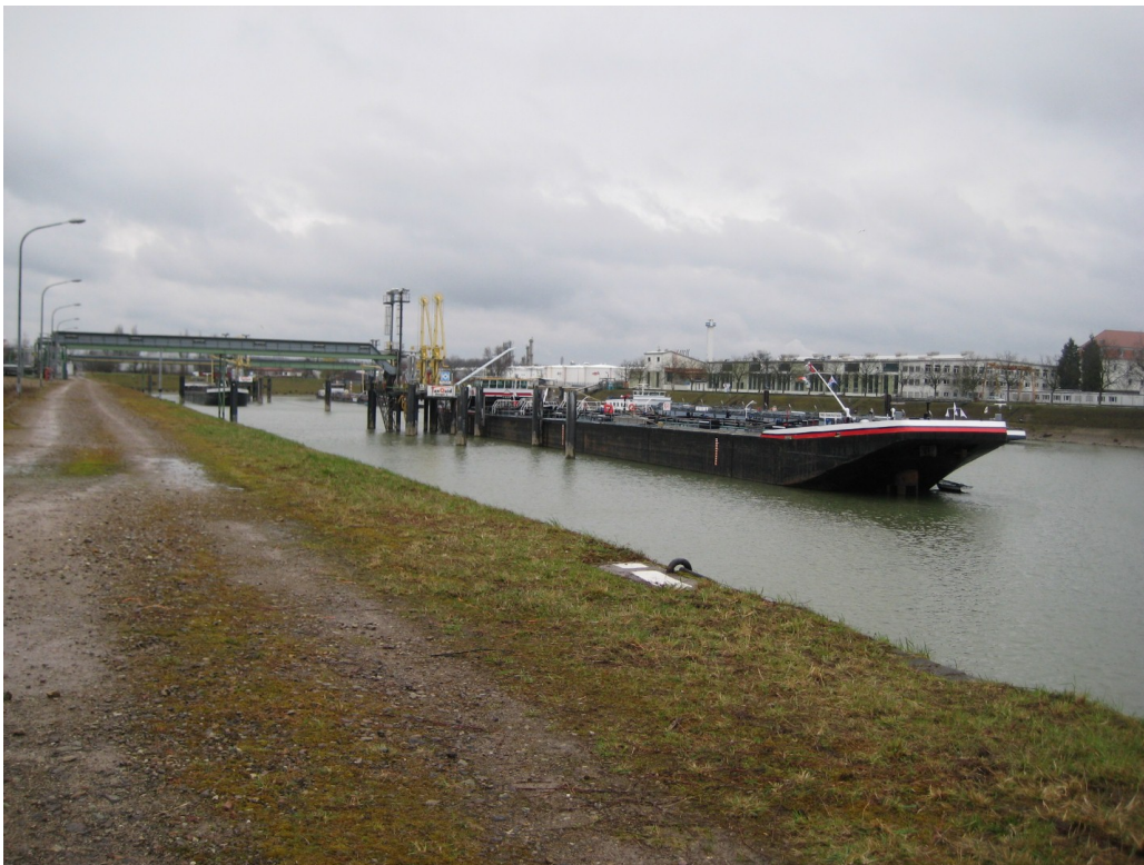
Fig.7: Modern 110 m tanker at the unloading station (Photo: C. Dahlhoff)
